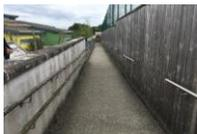
Ramps should have the following dimensions: 1.5m wide with a minimum unobstructed width of 1.5m.
