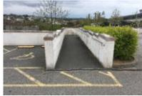
Install a further handrail on the ramp from the car park which currently only has one to ensure that there are handrails each side of the ramps.
